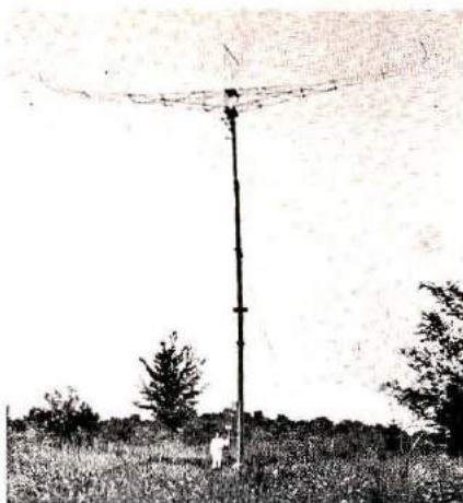
The first rotatable "8JK" antenna. It was built in 1937 for operation at 14 MHz.
